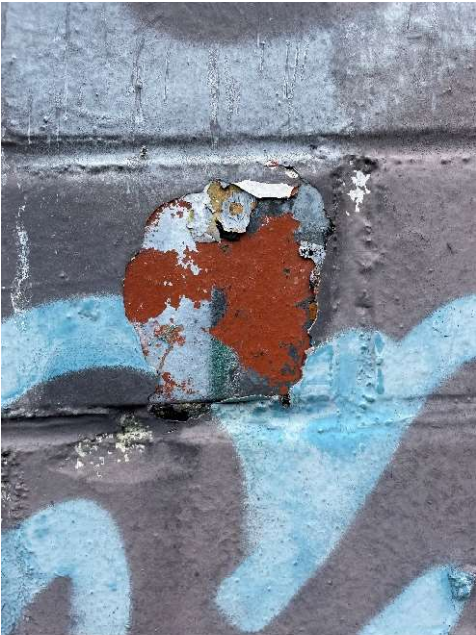
Do not overpaint graffiti, which is on top of damaged, earlier paint. The new paint will quickly fail.
