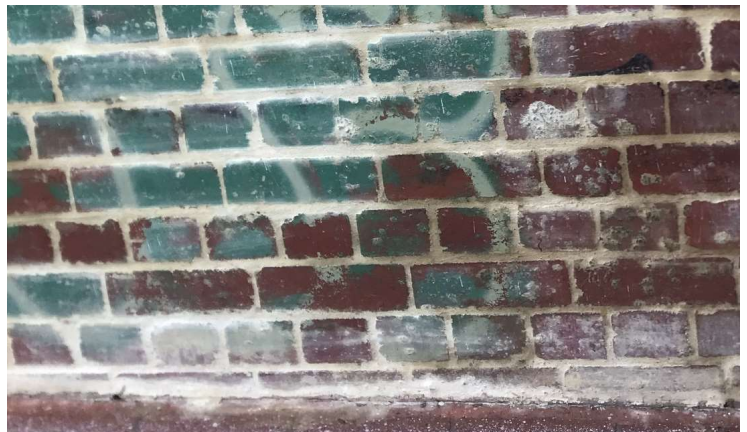
This wall was repointed before the graffiti was removed and the repointing was not done in accordance with the Heritage Technical Codes. This has not addressed the rising damp and left a thin layer of mortar covering the bricks and paint. It may not be possible to remove the graffiti as a result.
